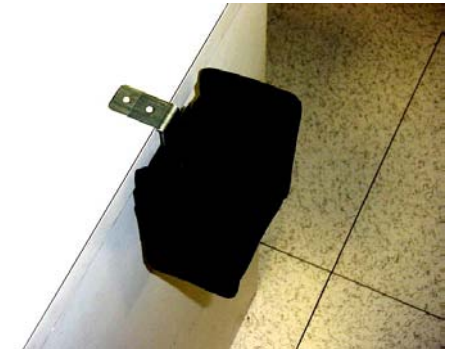
Figure 5 – Fixing HLS-8000 bracket on upper surface
